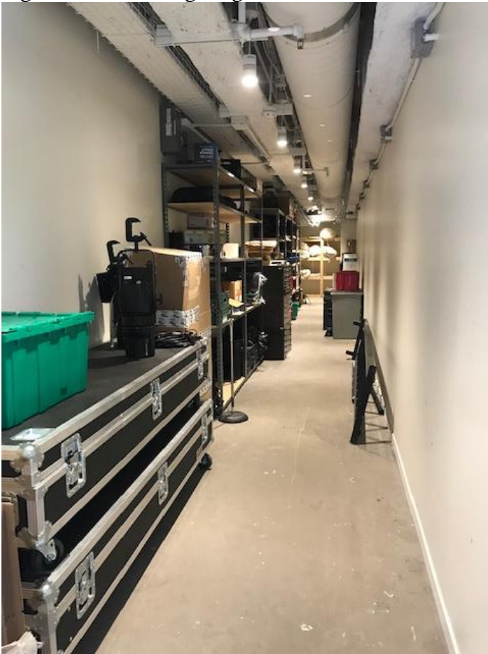
Figure 1: Theatre Lighting Closet
